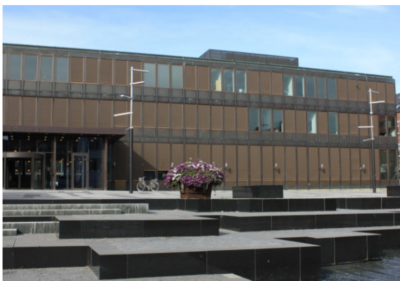
Guards at the service centre in Fredericia receive critical panic alarms on MOTOTRBO radios when employees press their panic buttons.
